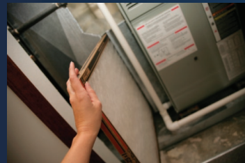
Indoor Air Quality Investigation
